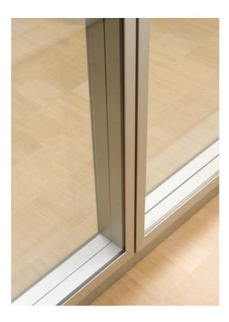
The supporting substructure consists of floor and ceiling-mounted profiles that hold supporting steel mullions. The glazed elements on both sides are single-pane or laminated safety glass panes sitting within aluminium frames and are inserted into the mullion construction. The wall thickness is 100 mm, or 125 mm where requirements for sound insulation and/or statics are higher.
